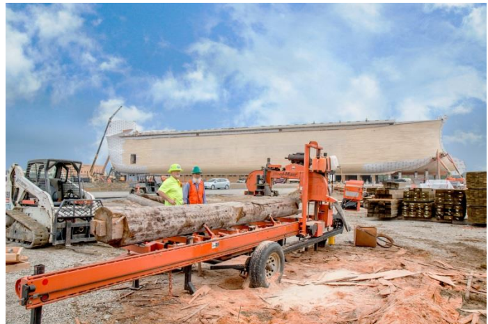
A Wood-Mizer portable sawmill onsite for additional construction needs.
